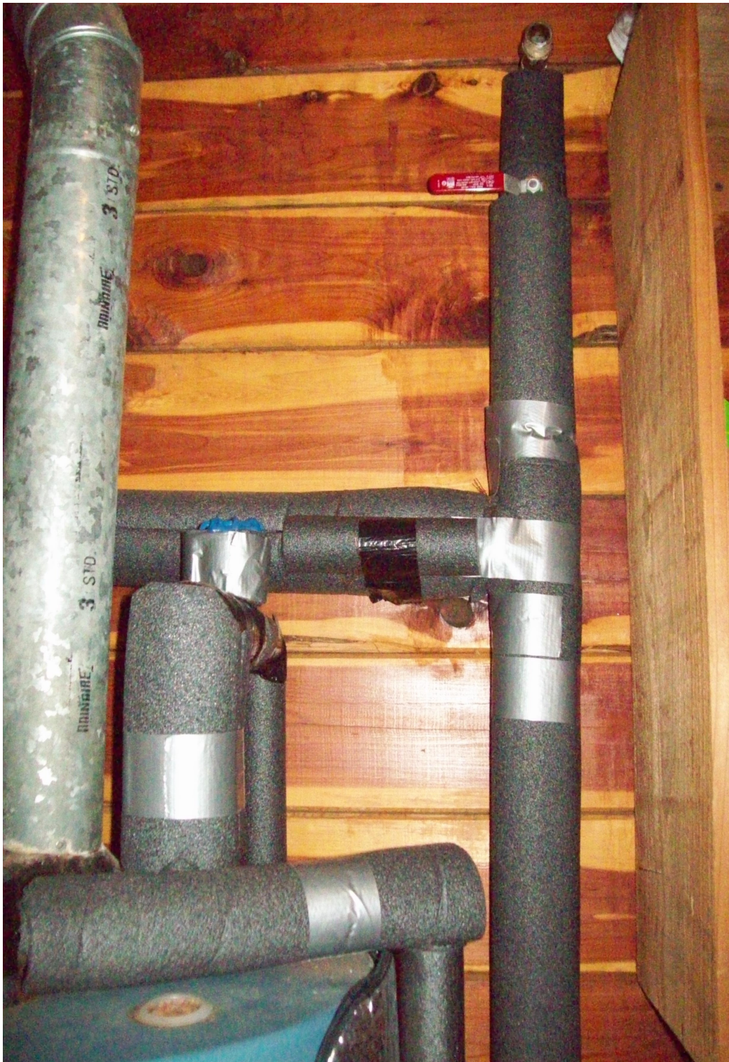
This shows the automatic air bubble remover (the fat line is the hot feed from the solar panel). The valve with the blue handle is the cold inlet and it remains untouched. Our valve which isolates the panel is covered here but it is positioned where the black tape is seen in the center of the picture.
